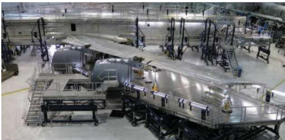
Instant UpRight design and manufacture a range of access systems for the aviation industry ranging from basic staging to full docking systems. We design and install both modular and fixed systems for every type and size of aircraft using heavy duty lightweight aluminium.
