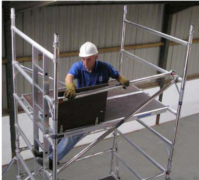
The 3T method was a significant step forward in mobile tower safety and when followed correctly, it ensures the operator does not stand on an unprotected platform which was one of the unsafe practises carried out prior to its implementation. The 3T method is arguably a straightforward and consistent process that does not vary depending on the make or configuration of a mobile tower which is obviously a significant safety, operational and training advantage.
