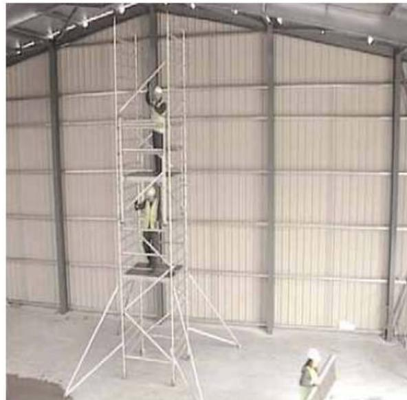
The second method of erection is the 'through-the-trap' (3T). This allows the person erecting the tower to position themselves at minimum risk during the installation of guard rails to the next level. It involves the operator taking up a working position in the trap door of the platform, from where they can add or remove the components which act as the guard rails on the level
