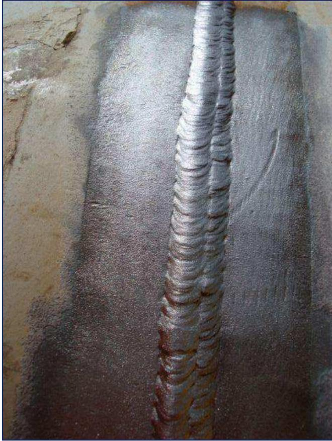
**Left:** This is an excellent view of a blast-cleaned weld, ready for application of the Zinga coating.
