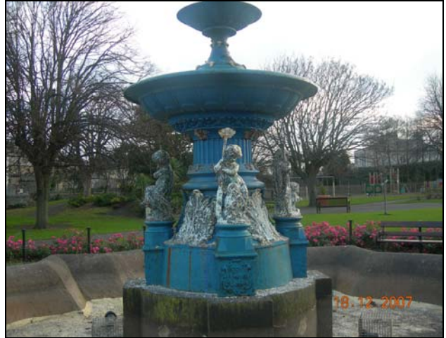
December 2007 - water turned off
