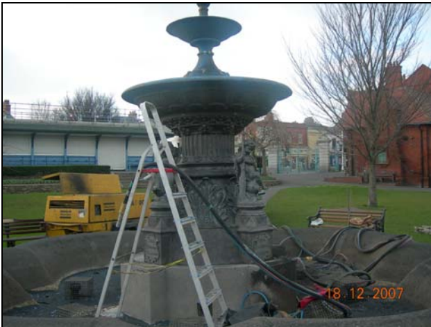
December 2007 – blast-cleaning to remove old paint
