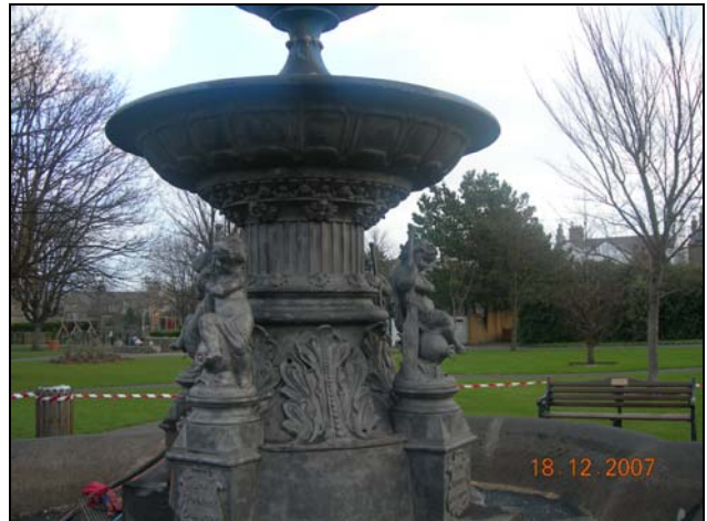
December 2007 - blast-cleaning showing fine details
