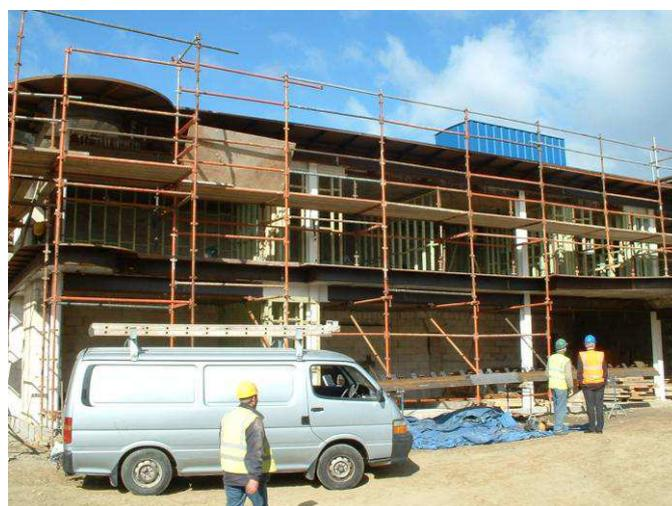
Above: A view showing the H-beams that were hidden by brickwork
