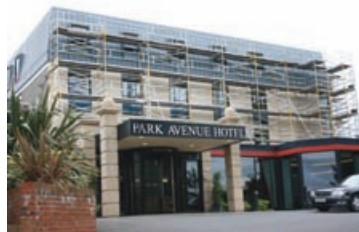
Ridgeway scaffolding at the Park Avenue Hotel, Belfast.
