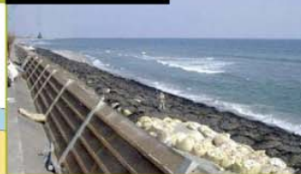
Works in progress
