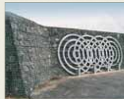
! Trapions™ form a sound barrier at the ECOS Centre, Northern Ireland. Constructed 1999.
