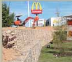
McDonalds, Chantier, France :: constructed 2004.
