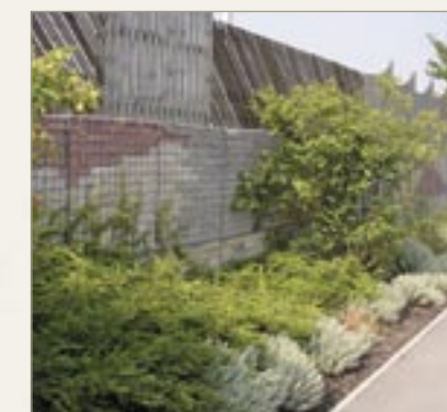
Shopping Centre boundary with concrete colour inserts. England, constructed 1998.
