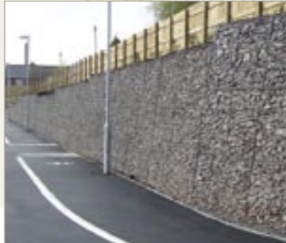
Gravity retaining wall at Europes largest Tesco superstore, Coventry, England. Constructed 2004.
