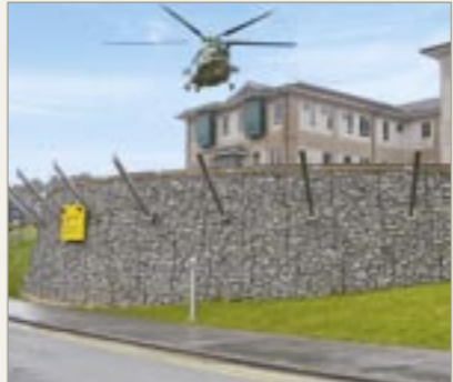
Gravity retaining wall supporting a helipad at Truro Hospital, England. Constructed 2004.
