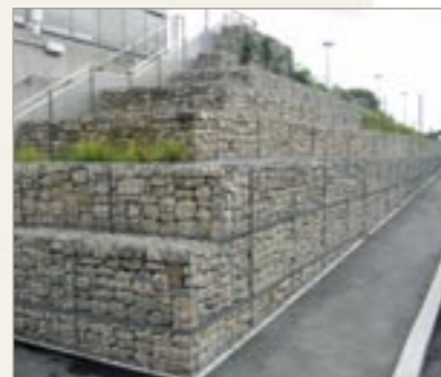
Retaining wall, Score Project, London, England. Constructed 2004
