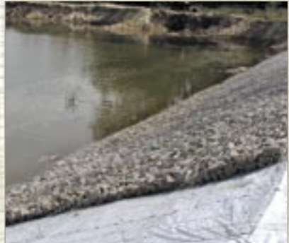
Shore protection using Weldmesh® Mattresses, Czeszow, Poland. Constructed 2005.
