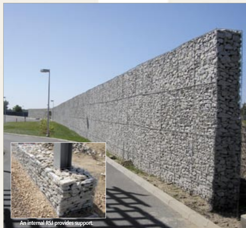
A free standing, internally supported perimeter wall provides strength and durability for the new Gillette factory in Lodz, central Poland. Constructed 2005.
