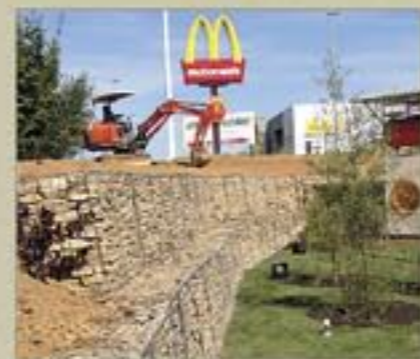
McDonalds, Chantier, France :: constructed 2004.
