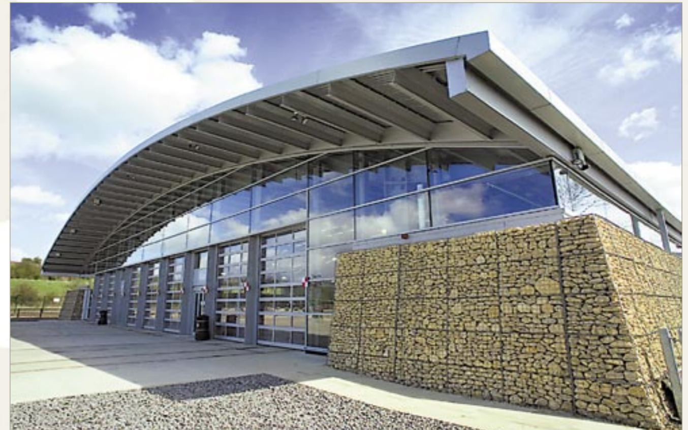
Locomotion Museum front entrance facade with Trapion™ walls and yellow limestone fill.
