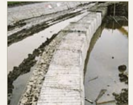
Concrete filled Bastion flood wall construction, Collier Street, Scotland. Constructed 2001.
