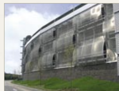
Free standing Trapions™ clad a multi-storey car park. Clarence Dock, Leeds, England. Constructed 2004.
