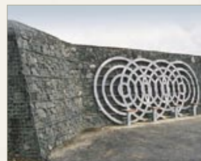
Trapions™ form a sound barrier at the ECOS Centre, Northern Ireland. Constructed 1999.
