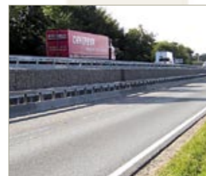
Highway application, A1 Kettering, England.
