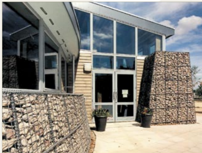
Earth Centre, England. An environmentally friendly development which took full advantage of Trapion™ walls with a graded, crushed concrete fill. Constructed 2000.
