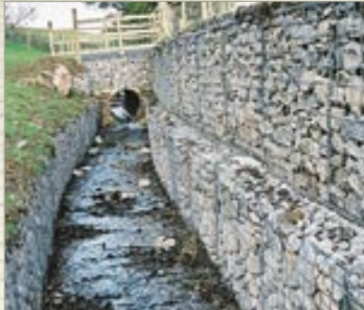
Channel lining constructed with Gabions and Mattresses, Graigfechan, Wales. Constructed 2000.
