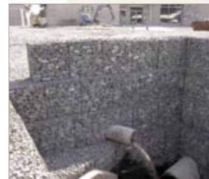
Gabion as an integral part of a drainage structure. Constructed N.Ireland, 2002
