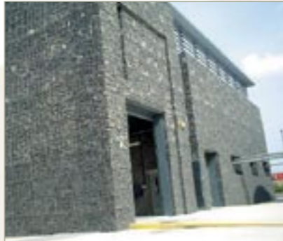
Architectural cladding to Duncrue Scrubber Water Treatment Works, Belfast, N. Ireland. Constructed 2004.
